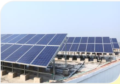
1. Solar generation Installation of Solar panels
